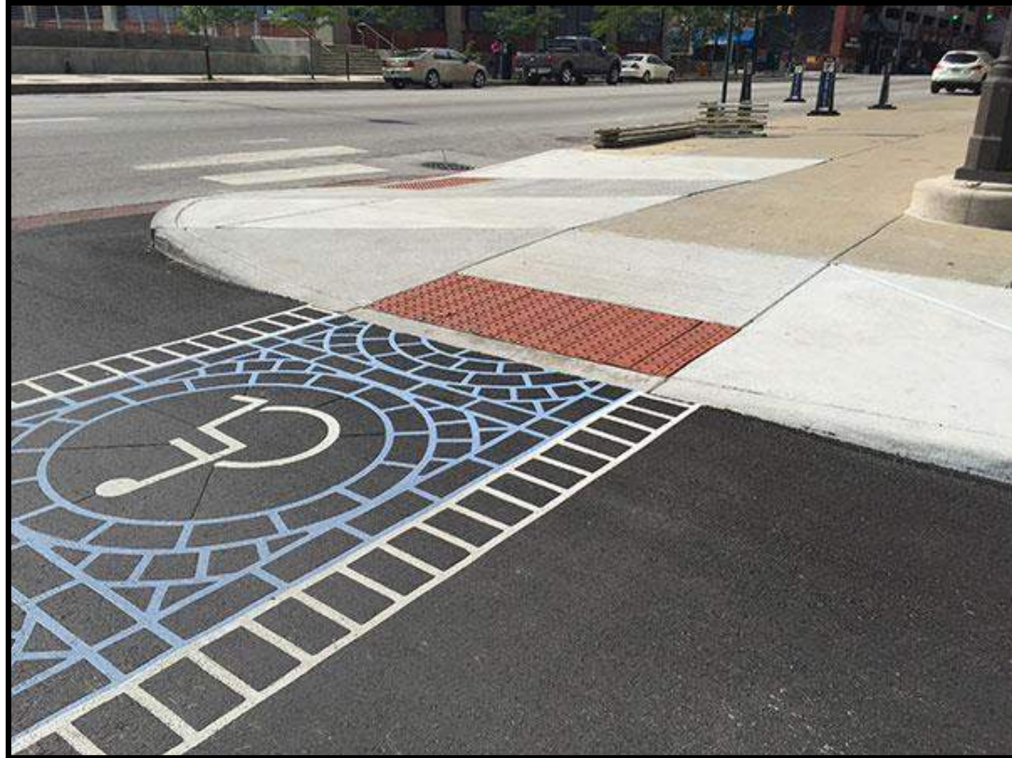
ADA SITE IMPROVEMENTS
