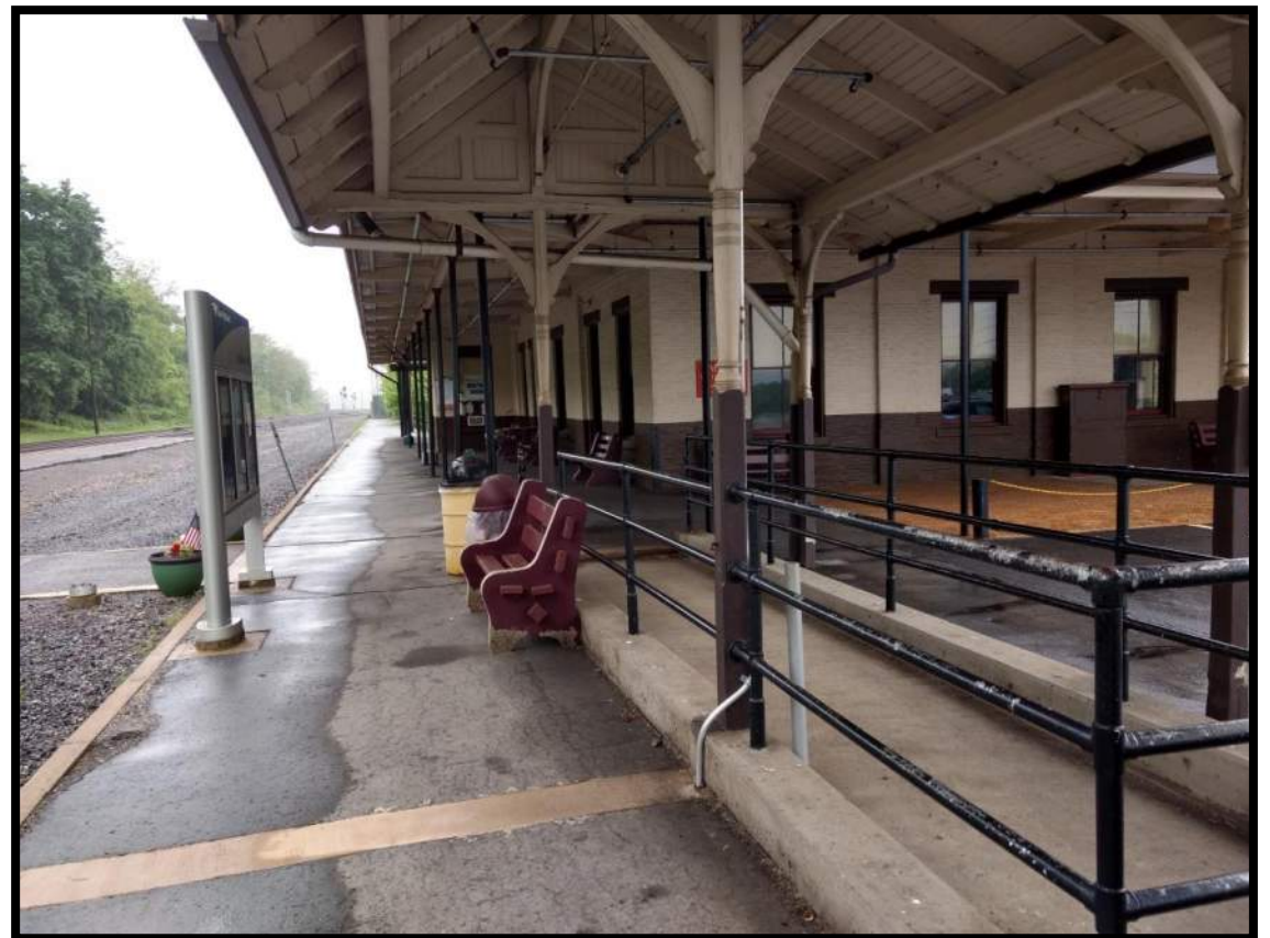
VIEW OF STATION BUILDING AND CANOPY LOOKING NORTHWEST
