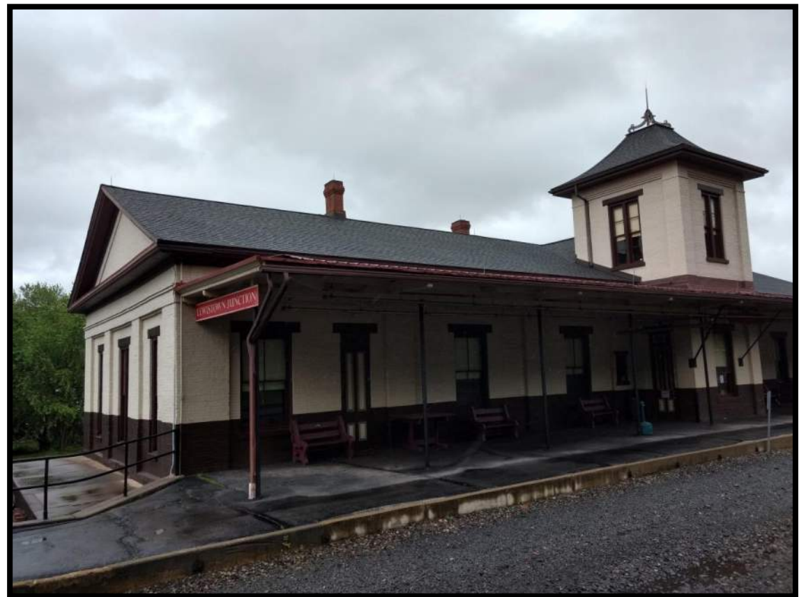
VIEW OF STATION BUILDING LOOKING NORTHEAST
