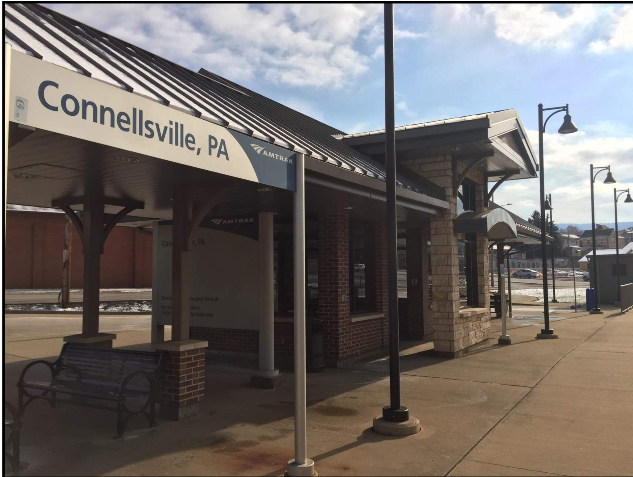
AMTRAK CONNELLSVILLE, PA WAITING BUILDING AND CANOPY
