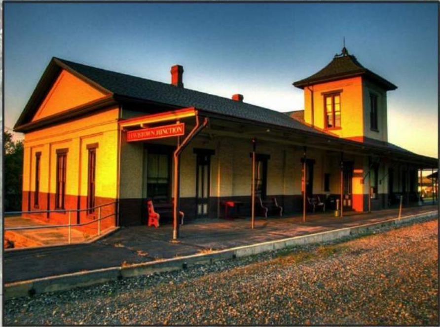
View of existing Lewistown Junction Station building.
