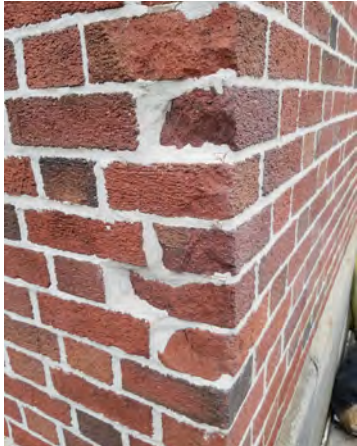
DAMAGED BRICK
