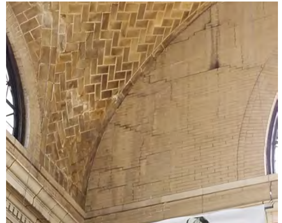
CORNER OF VAULTED CEILING IN MAIN HALL WAITING AREA
