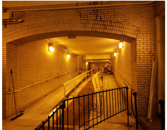
ACCESSIBLE RAMP IN ACCESS TUNNEL
