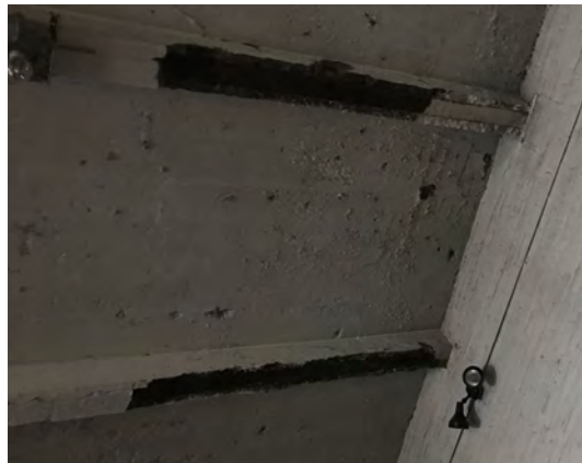
STEEL BEAM IN CONCRETE-BAGGAGE/EXPRESS BUILDING
