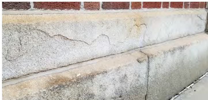
SUGARING STONE AT GRANITE BASE
