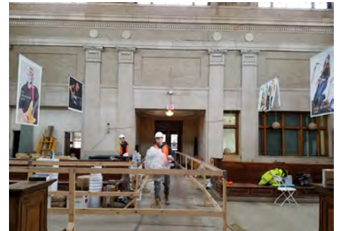
EAST INTERIOR WALL WITH OLD TICKET WINDOW
