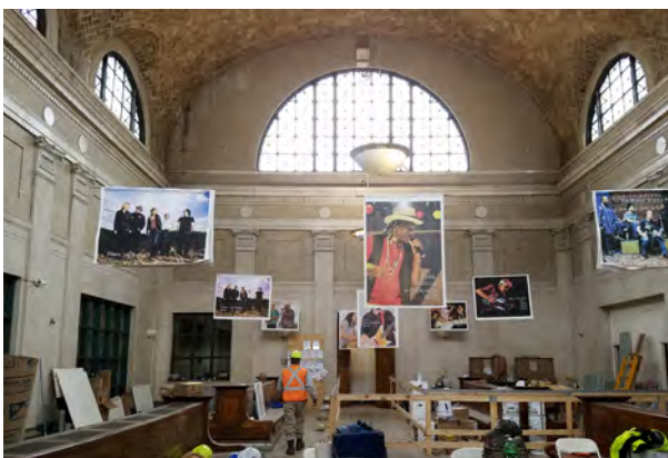
MAIN HALL WAITING ROOM LOOKING NORTH
