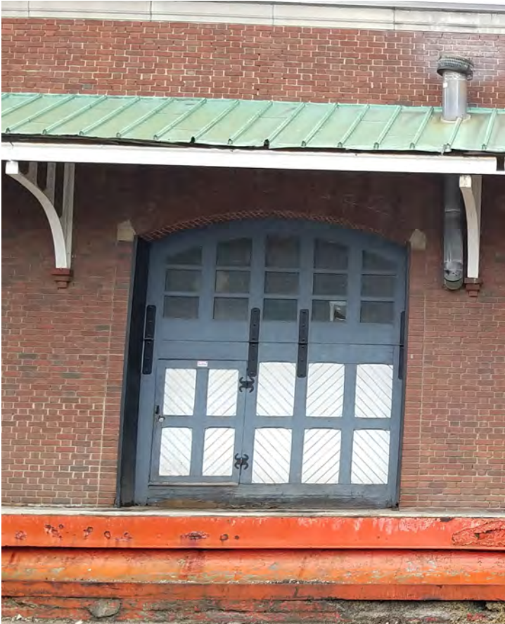
VERTICAL FOLDING GARAGE DOOR
