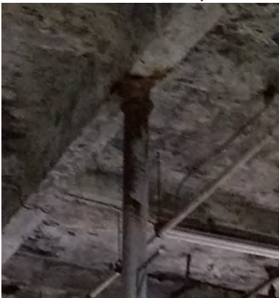
COLUMN IN BAGGAGE/EXPRESS BUILDINGS
