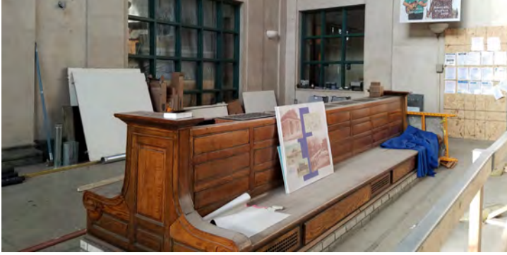
INTERIOR WALL MAIN HALL WAITING ROOM
