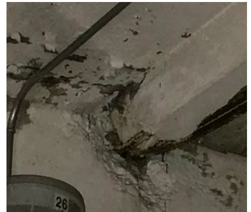
REINFORCED CONCRETE BEAM IN GARAGE BUILDING
