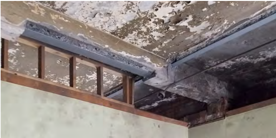
SECOND FLOOR CEILING - BEAMS ENCASED IN CONCRETE
