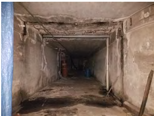
ABANDONED BAGGAGE TUNNEL
