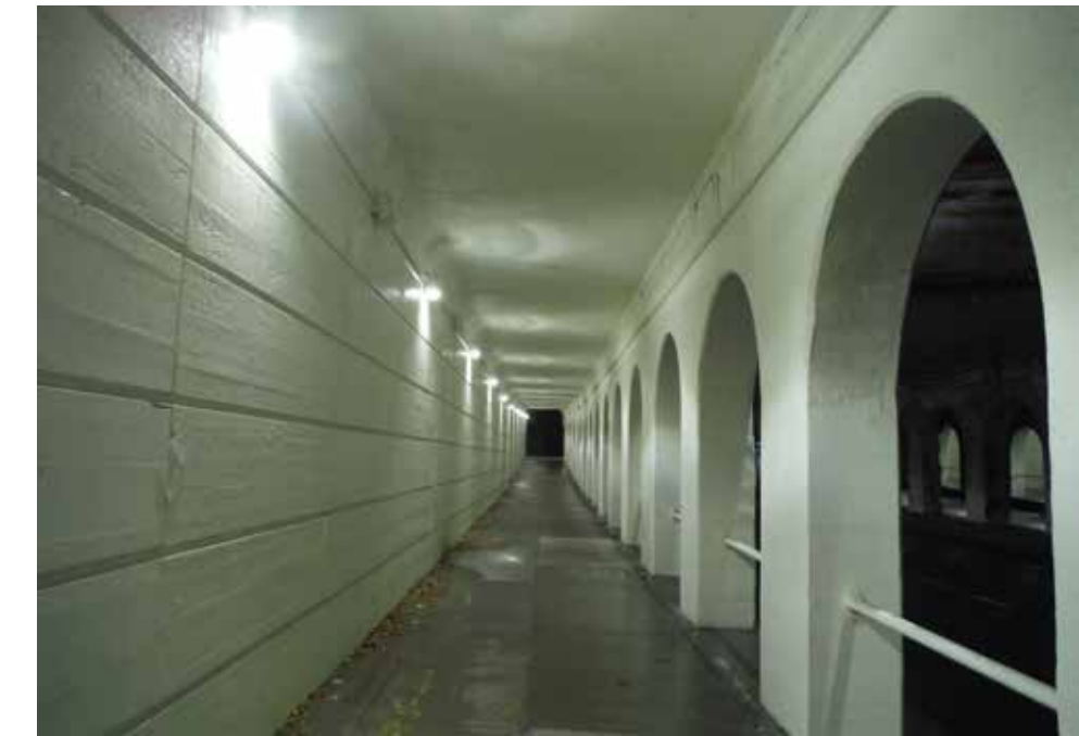
Market Street Underpass Improvements
