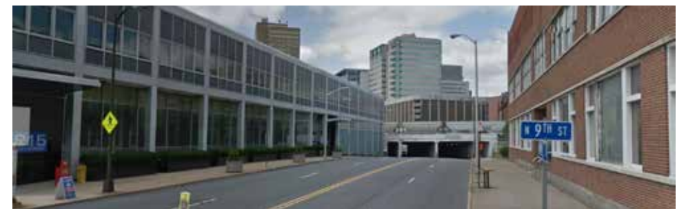
Existing Conditions East of Railroad Tracks
