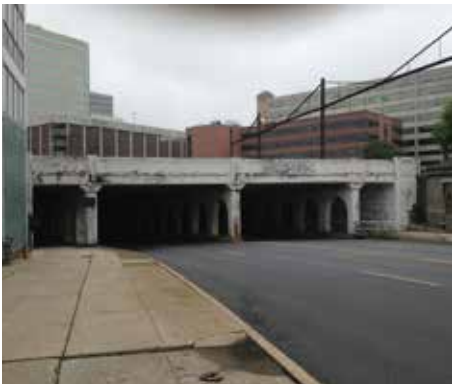
Market Street Underpass
