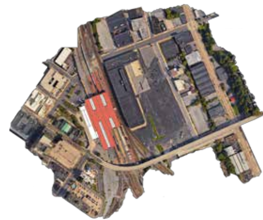
Phase 1 HTC Station Rehabilitation
