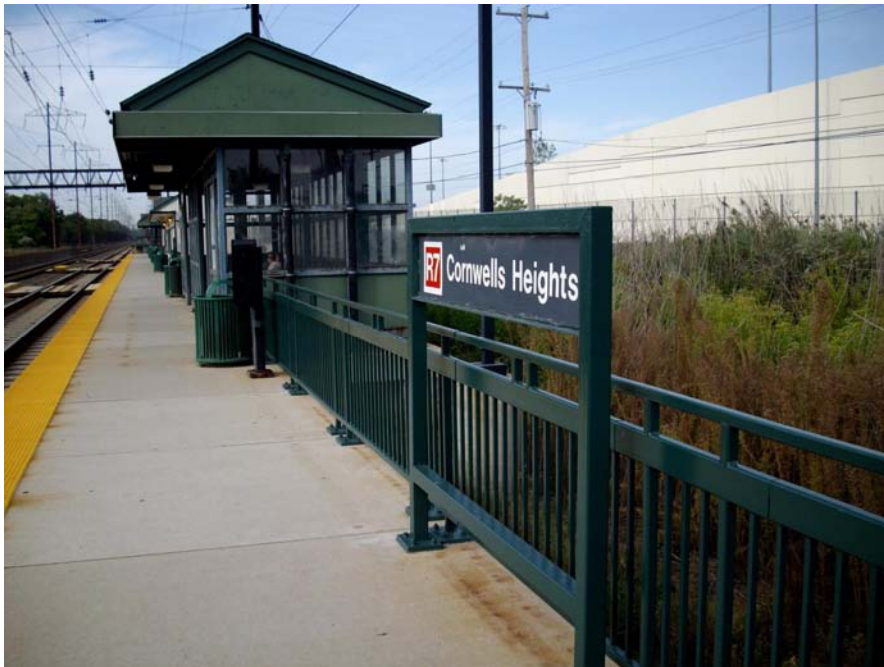
Figure 3: Existing Cornwells Heights, PA Station
