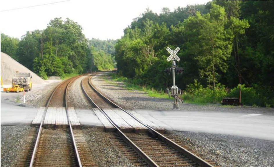
Figure 14: Typical Grade Crossing on the Pennsylvanian
