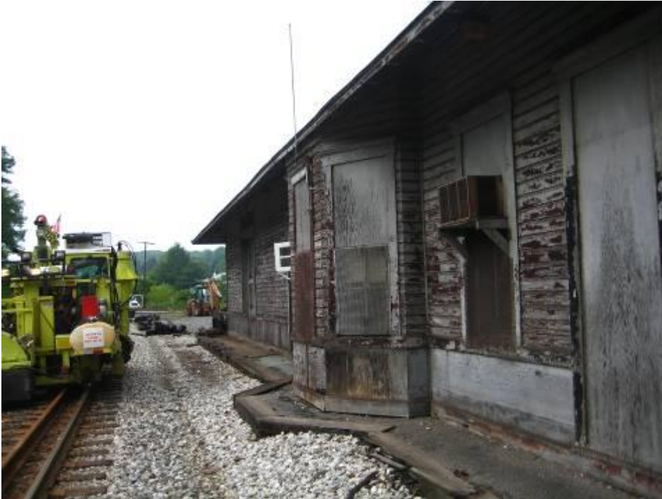
Figure 17: Existing Rockwood, PA Station (owned by CSX)
