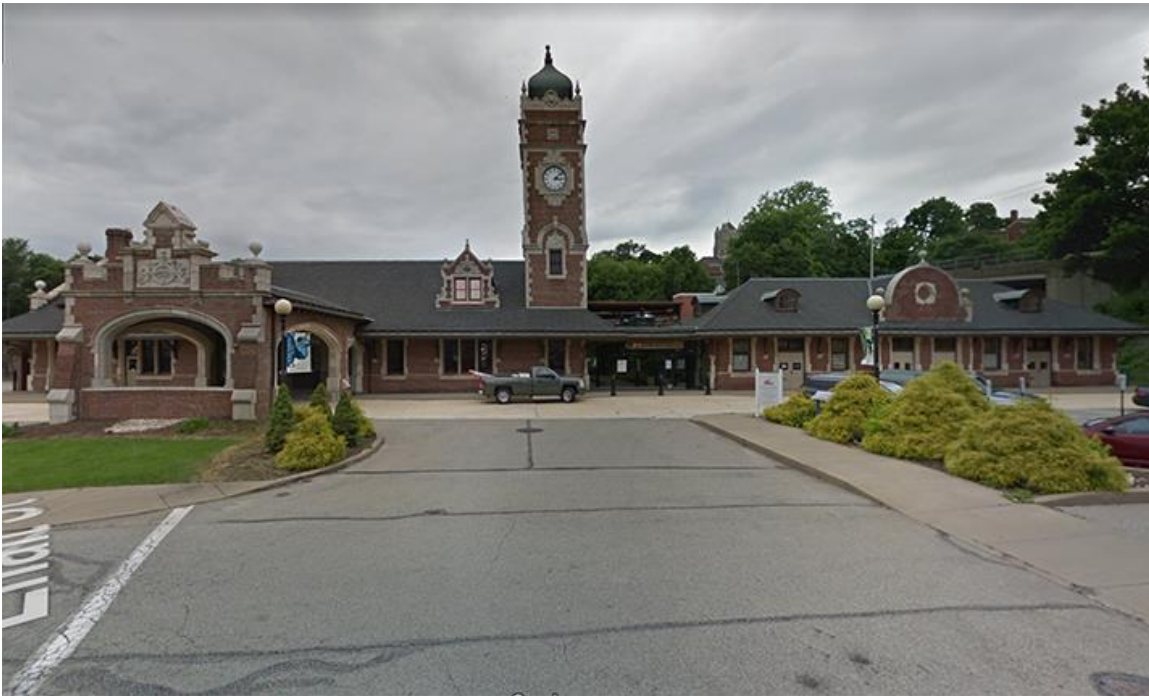
Figure 9. North-Facing Street View of Greensburg Station Building
